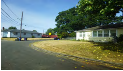
Photo 3.3.5. Attached housing, Lincoln Heights District
